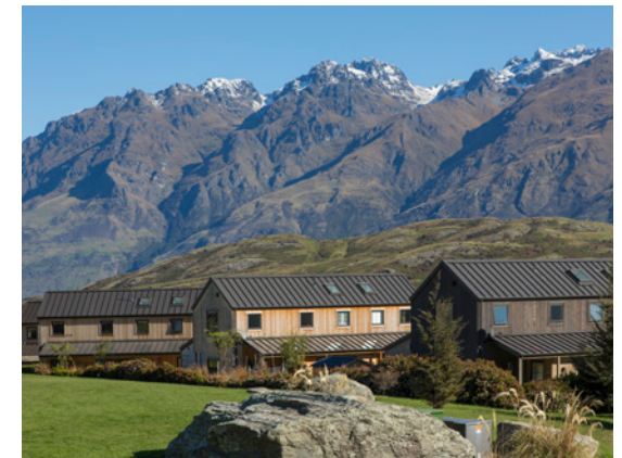
Lean-to roof subservient to the principal gable form.
