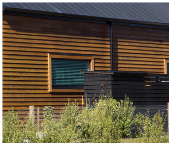
Site utilities and service area screened with material to match cladding
